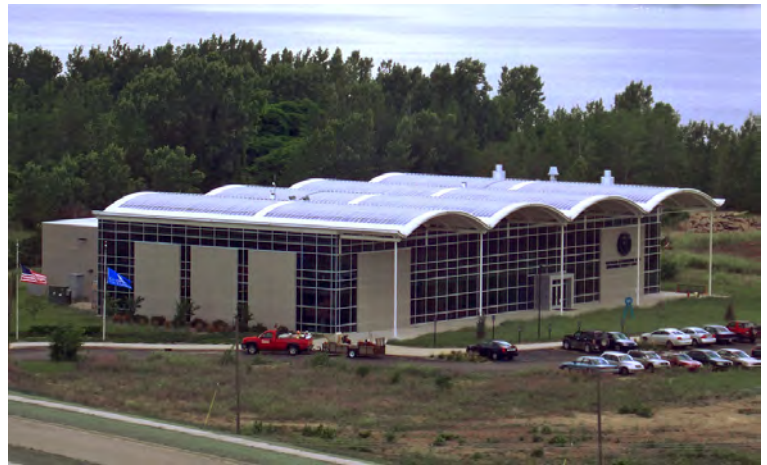
Michigan Alternative and Renewable Energy Center (30kW) Grand Valley State University, Muskegon, MI
